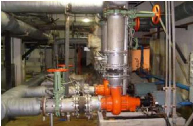
Installation of pumps
