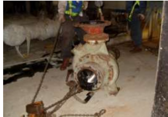
Heat exchange pump
