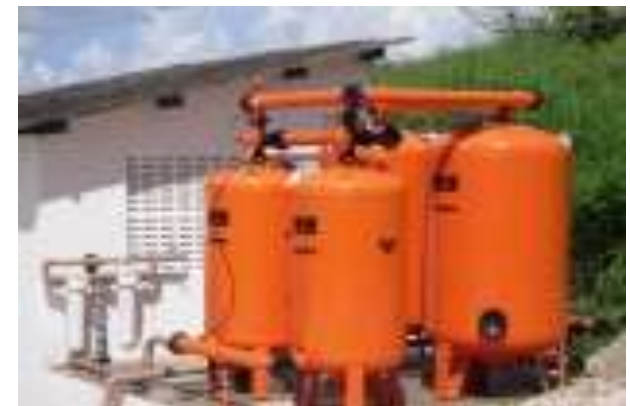
Small and modular water treatment plant
