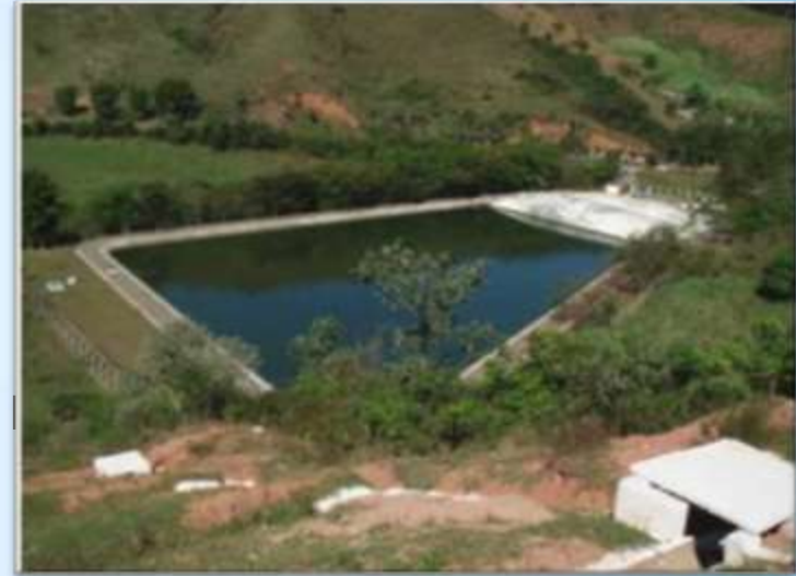
WWT Silveiras plant
