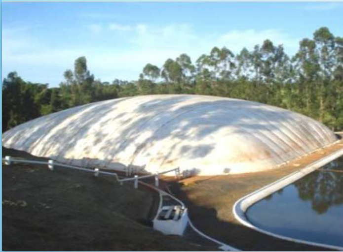
WWT Auriflama plant
